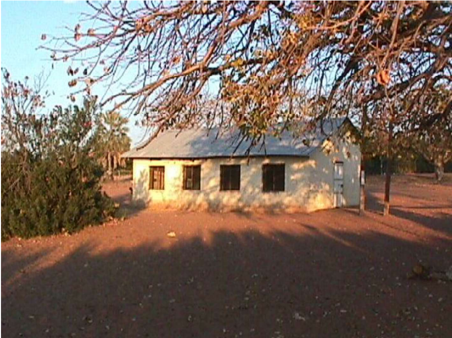
Figure 279: This former Primary School in Sauyemwa – which later moved to the premises of the Sauyemwa Combined School – traces its existing to an initiative of Makaranga. The foto was taken in 1999.
